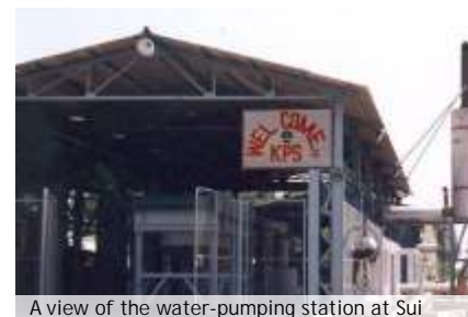
A view of the water-pumping station at Sui
